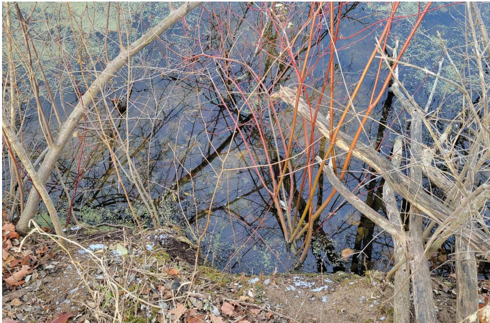
Upstream Side of Seepage Location
