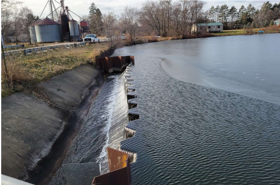
Weir Alignment Looking West
