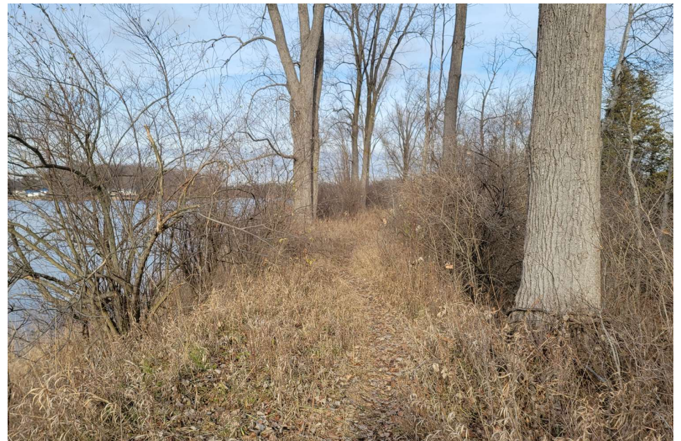
Looking North from Auxiliary Spillway
