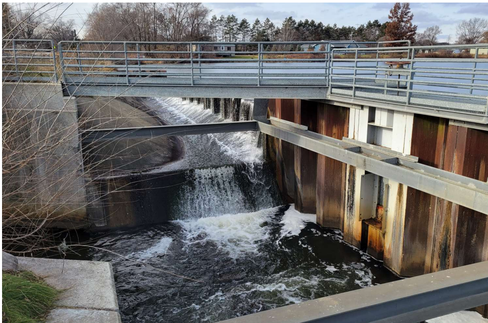
Looking West at Dam Structure
