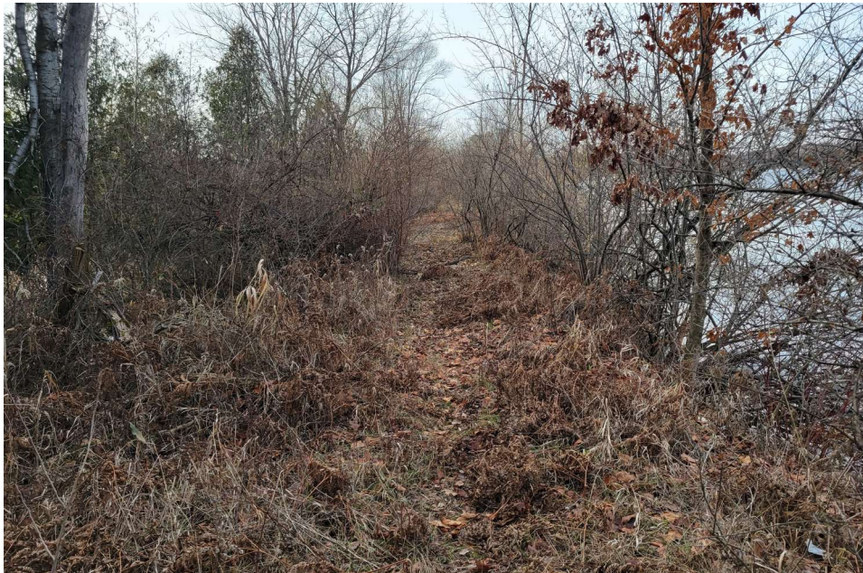
Eastern Portion of Embankment
