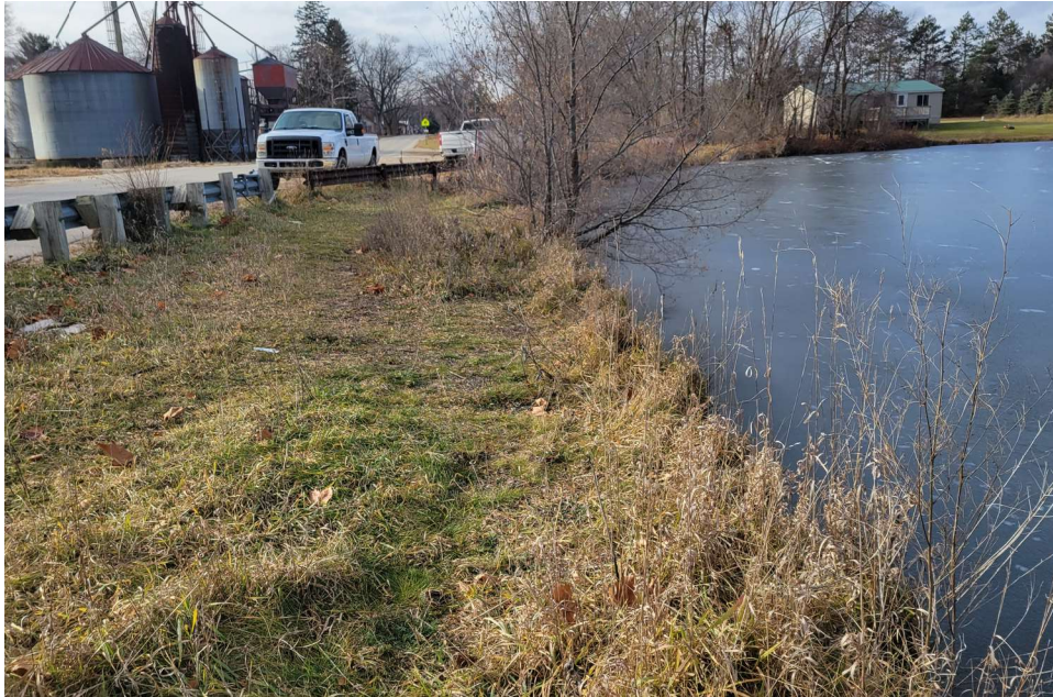
Looking West Along Western Embankment
