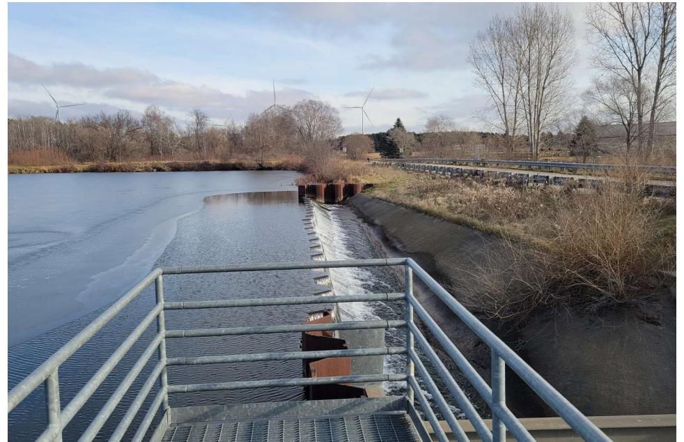
Weir Alignment Looking East
