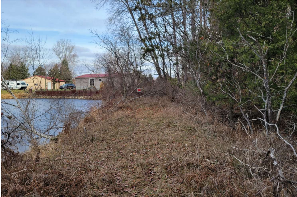
Farthest Eastern Part of Embankment
