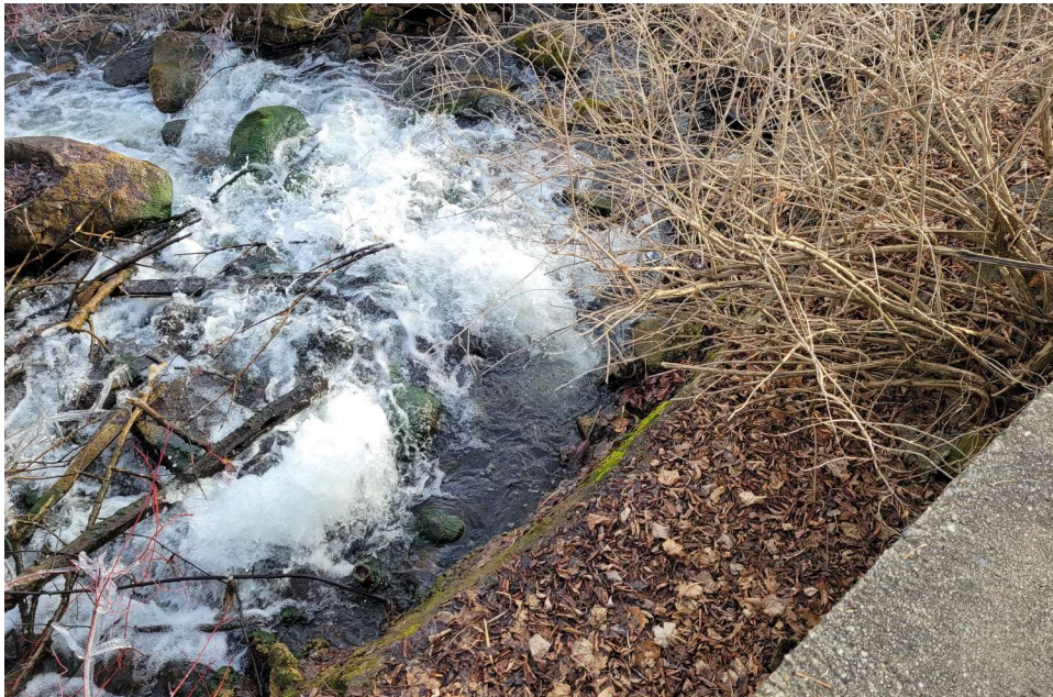
Cold Water Discharge Downstream of Auxiliary Spillway
