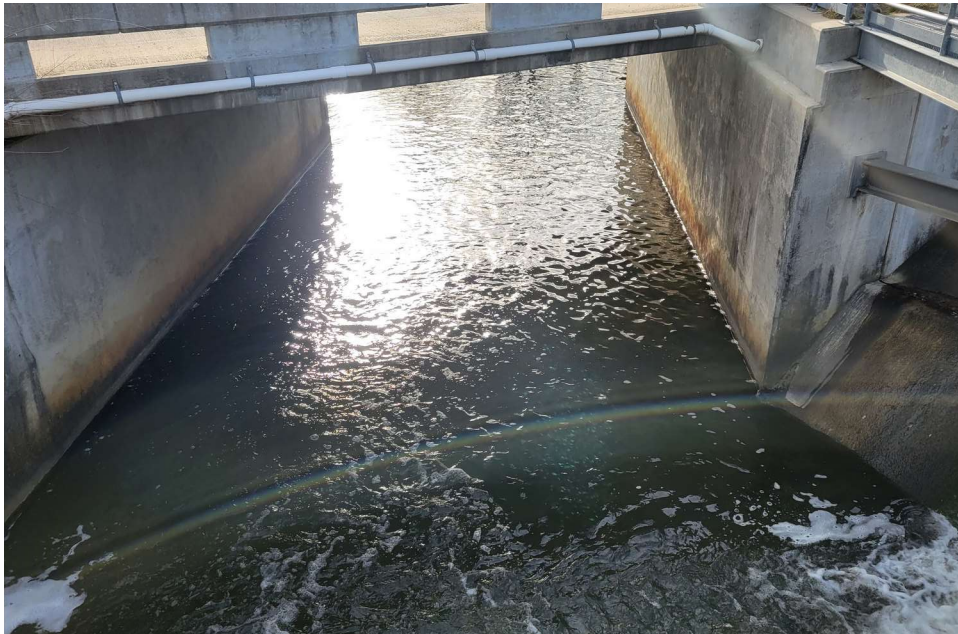
Concrete Condition through Outlet Channel
