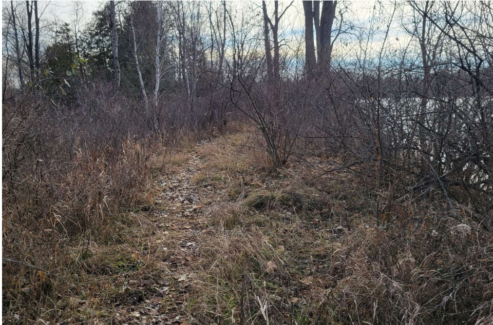
Looking Southwest on Eastern Embankment
