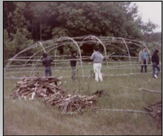
Constructing a lodge
