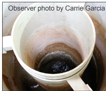
Observer photo by Carrie Garcia A recarbonation tank like the one shown above allows carbon dioxide gas to enter the water and help reduce the pH levels in the softened water.
